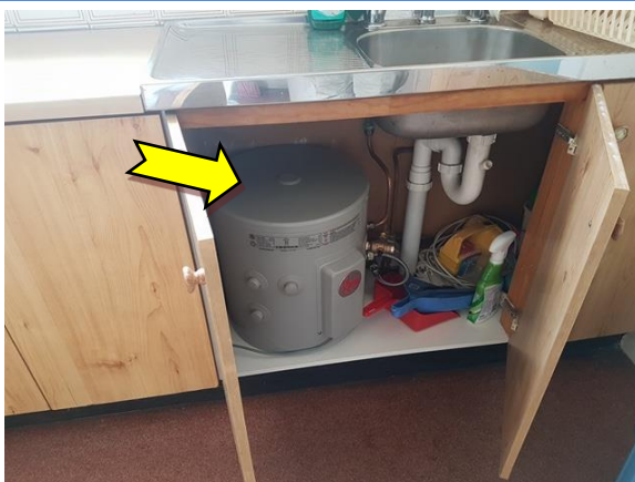
Photo 11. Interior, ground level, kitchen, hot water heater – suspected SMF internal insulation.
