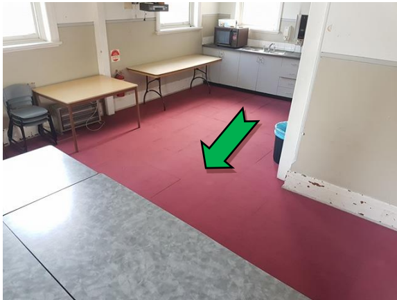
Photo 7. Interior, ground level, community room, beneath carpet, red floor covering – assumed non asbestos-containing floor tiles.
