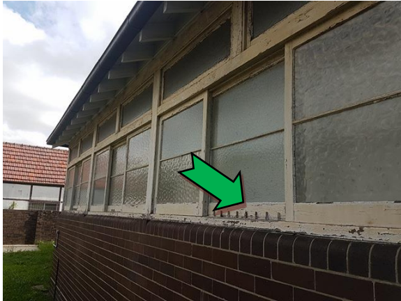
Photo 1. Exterior, throughout, window frames – non asbestos-containing window caulking.
