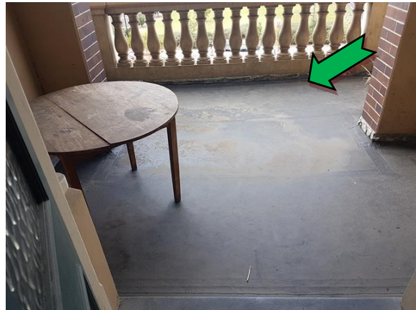
Photo 4. Interior, level 1, balcony, waterproof membrane – suspected non asbestos-containing bituminous material.
