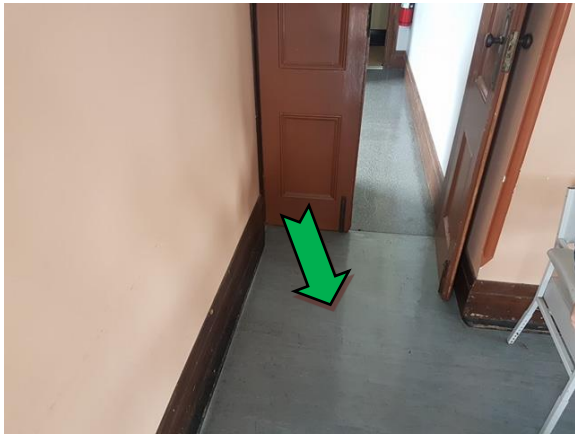
Photo 3. Interior, level 1, hall, grey floor coverings – suspected non asbestos-containing sheet vinyl.
