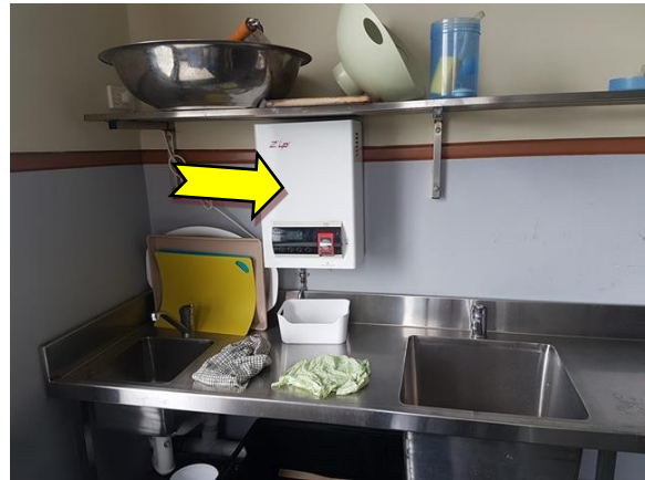
Photo 10. Interior, level 1, kitchen, hot water heater – suspected SMF internal insulation.
