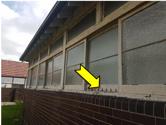
Photo 15. Exterior, throughout, window frames – cream upper coloured paint systems.
